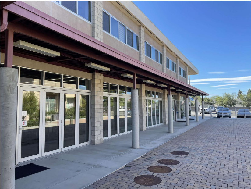
WESLEY CENTER - EXTERIOR VIEW FROM COURTYARD
