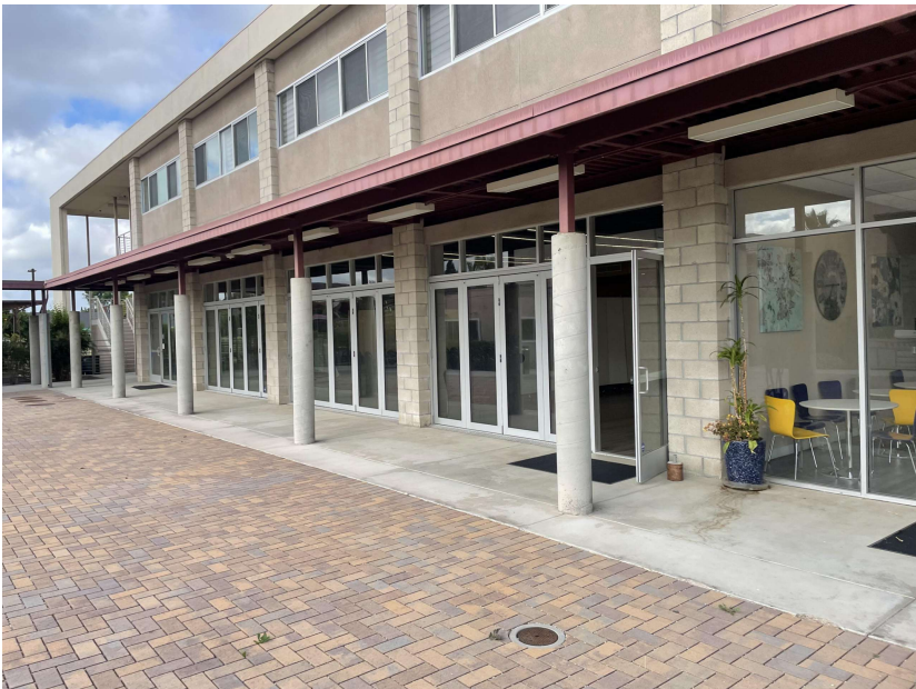
WESLEY CENTER - EXTERIOR VIEW FROM COURTYARD
