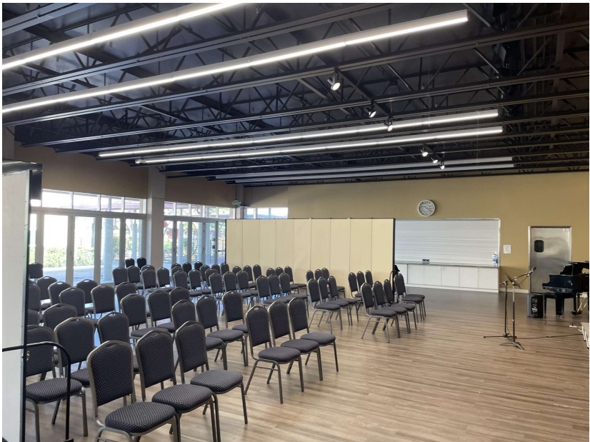
EXISTING MULTI-PURPOSED AREA FOR ADHC USE
