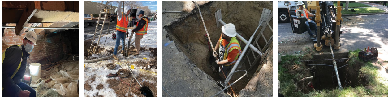
Field Identification and Replacement of galvanized and lead service materials
